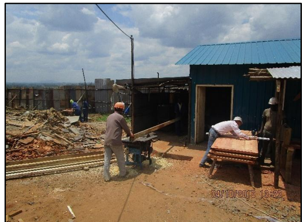
are itemised and summarised in table 9 below Figure 17: onsite Carpentry workshop, Notice man operating machine without personal protective gear
