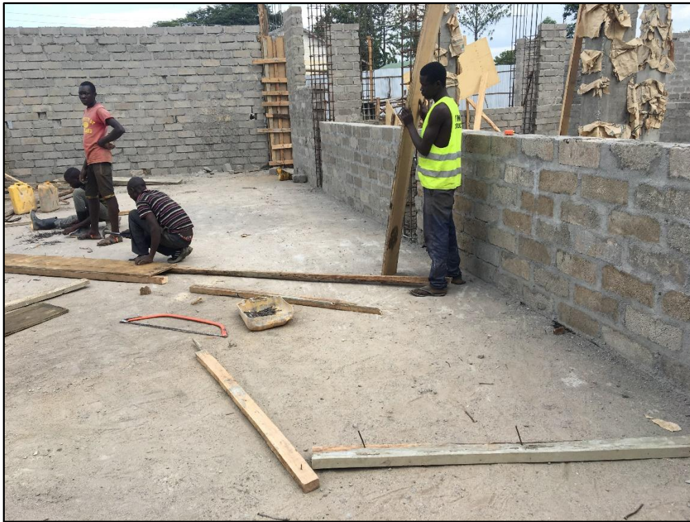
Figure 308: Workers carry out works without proposal protective gear, Notice the gentleman is a reflector Jacket donning slippers, operating right next to a timber piece with protruding nails, this constitutes a health and safety risk to the worker.
