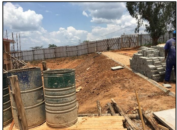
Figure 15: Unprotected Embankments
