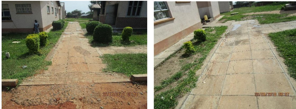
Figure 61: Failure along the side walk to kitchen
