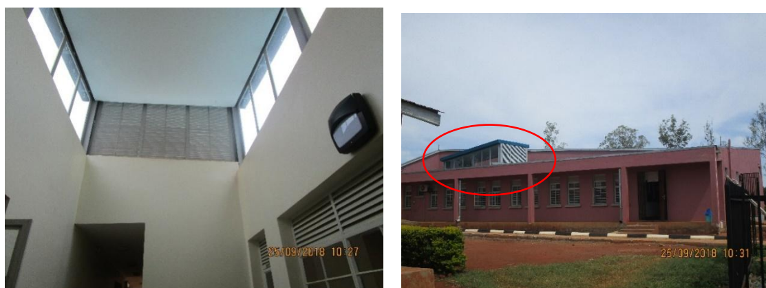
Figure 38: Roof design to allow for effective ventilation and lighting
