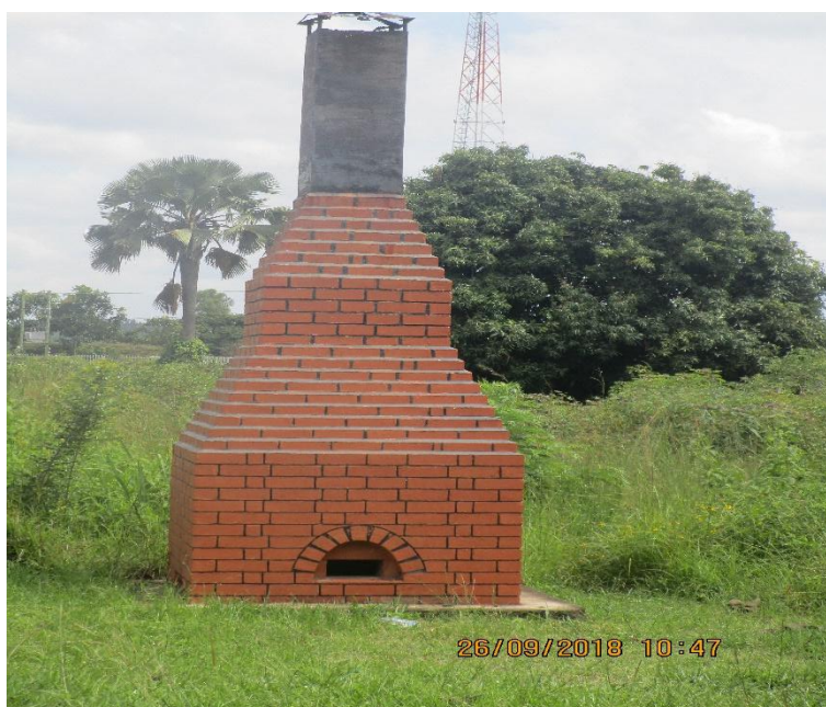
Figure 66: Incinerator constructed under additional works to the project
