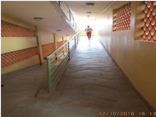
Figure 8: Ramps for access for Persons with disabilities
