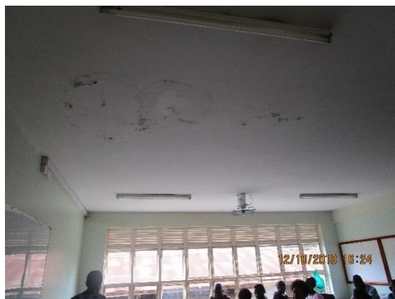
Figure 14: Leaking roof
