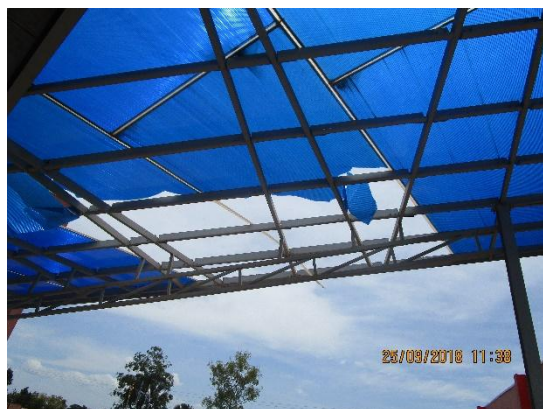
Figure 41: Failure on the roof of the pergola
