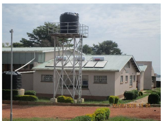
Figure 57: Solar water heater on dining hall roof
