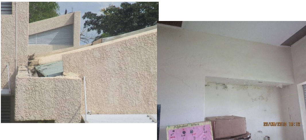
Figure 62: Rehabilitated roof still experiencing leakages
