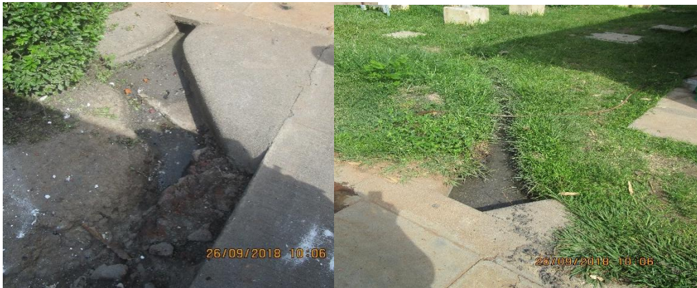
Figure 64: Blockage of kitchen waste water drain
