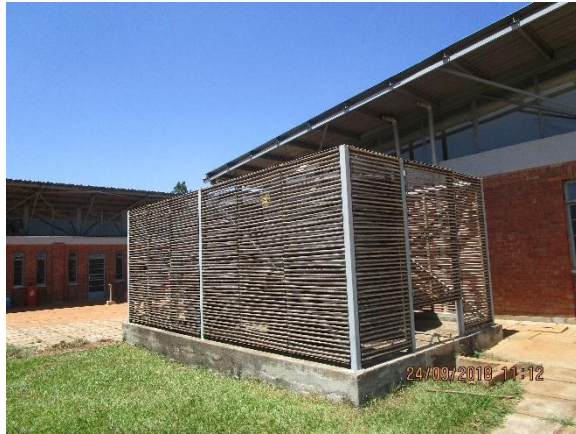
Figure 33a&b: Use of bamboo as cladding around the rain water tank
