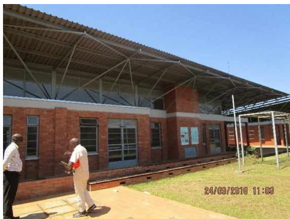
Figure 26: Roof design to allow for natural lighting
