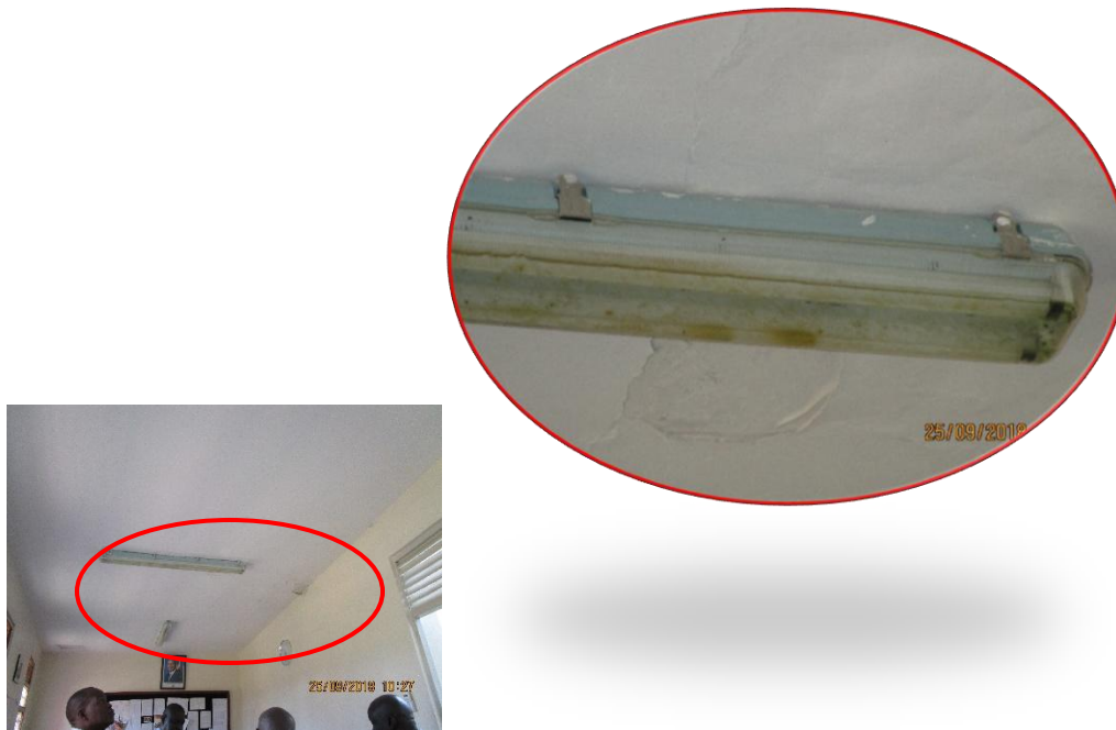
Figure 42: Signs of leakage on the roof
