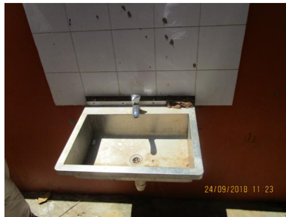
Figure 34: Broken sink pan at the new Male toilets
