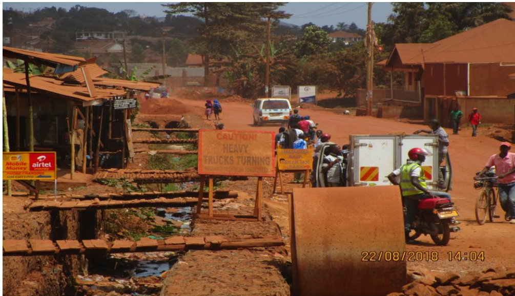
Figure 11: Poorly maintained accesses culverts on Namasuba-Ndeje-Kitiiko Road
