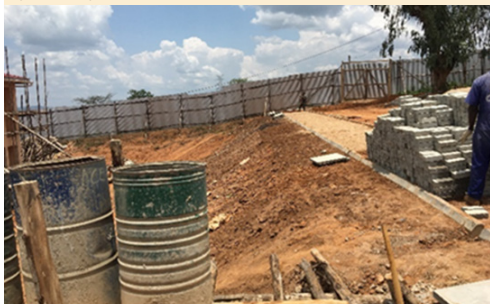
Figure 18: Unprotected embankment (HEST)
