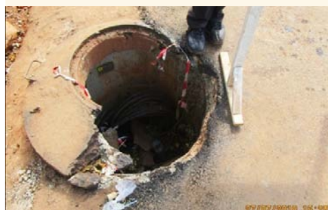
Figure 17: Unsecured service viaduct on St.Noah Nfuufu
