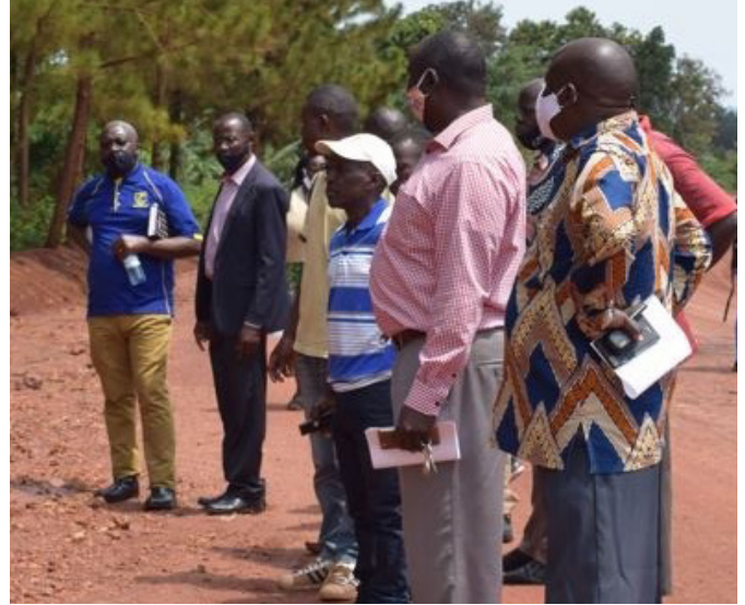
Site inspection of Busoga Mwiri college road construction works as part of independent review, June 2021.
